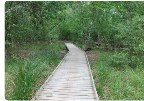
8 Boardwalks In some areas where the ground is prone to retaining moisture, boardwalks will maintain an accessible footpath throughout. This will use recycled plastic where possible and be accessible for wheelchair users and pushchairs.
