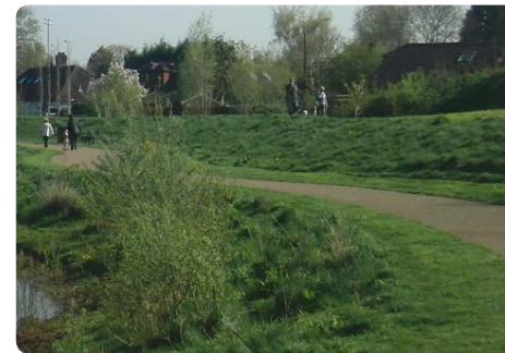
10 Bunds The use of bunds / embankments will be carefully located throughout the project area to help protect adjacent properties from flooding.
